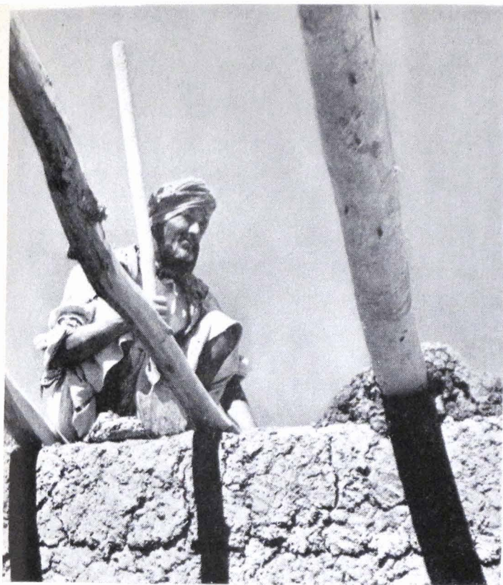
Left: Master-builder Shireen "the Sweet" placing beams for the roof of Jacques' new house. (See page 128.)
